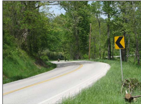
Typical Corridor View along KY 715
